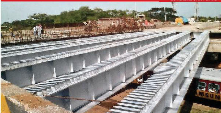
Composite Steel Girder
